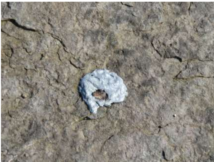
Figure 11 Poured lead shore-fasts at Barr'd Island Point
