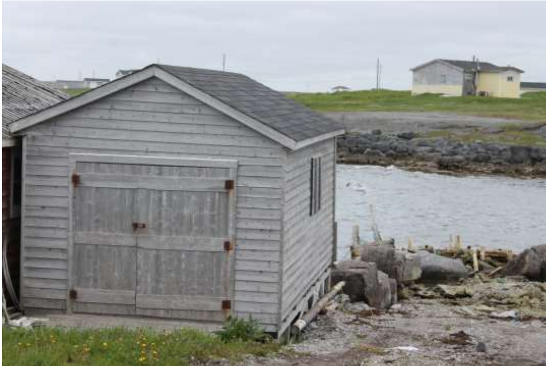
Figure 14 Clapboard shed, still in use.
