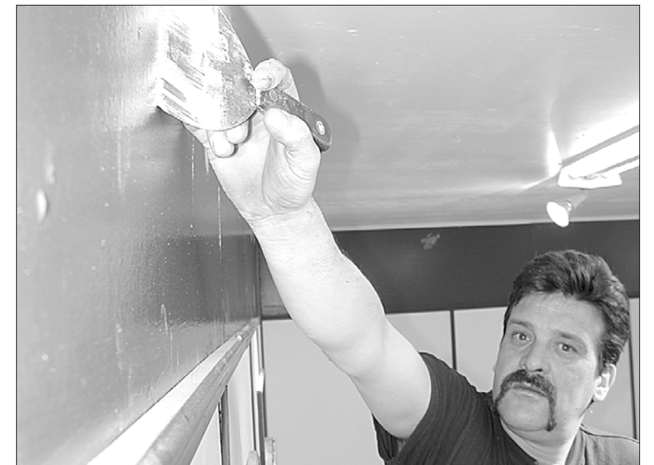
Improvements to the Great Brehat community hall were nearing the final stages in January as workers added some of the finishing touches. The 14-week project, funded by ACOA and administered by St. Anthony Basin Resources Inc., included the installation of new windows, siding, floors, ceilings, walls and pipe. Lorne Carter is shown applying plaster to touch up spots on a wall.
