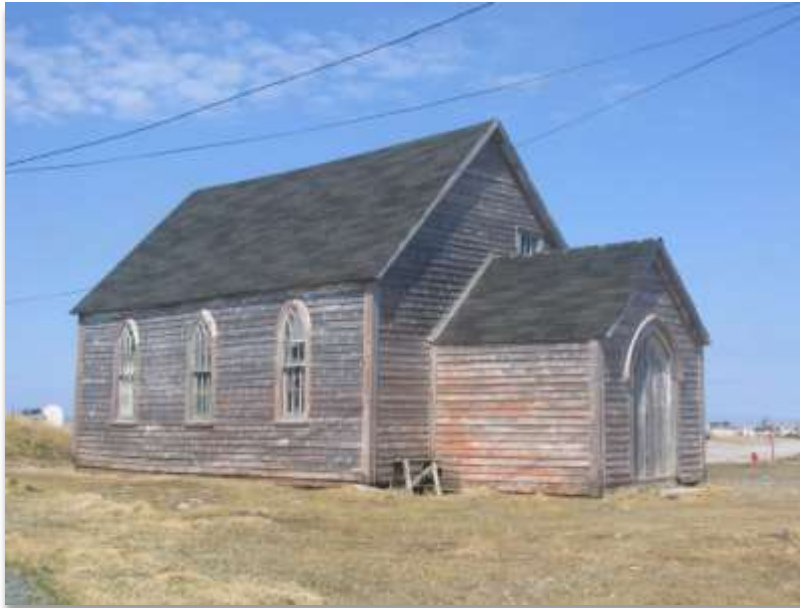
Figure 1 The old Methodist Church at Cook's Harbour has aged gracefully over the years
