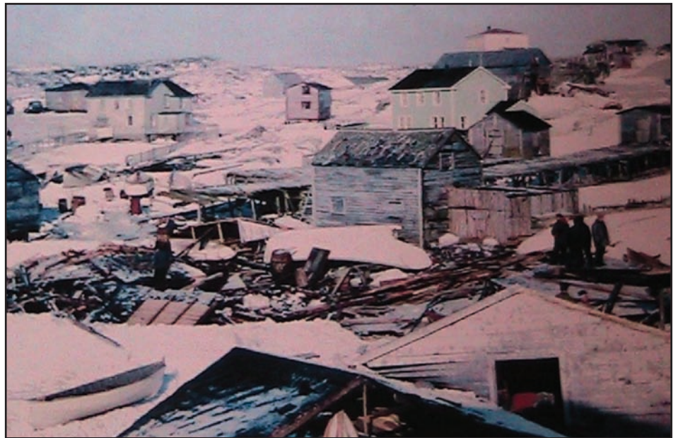
John Pilgrim's father is one of three men (seen to right of picture) surveying the wreckage of stages and breakwaters
